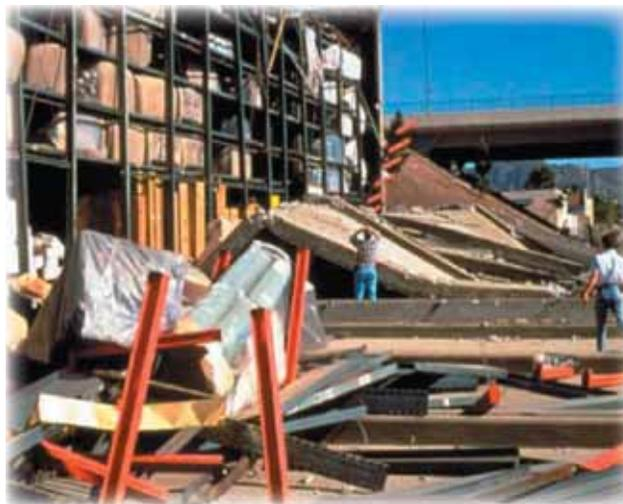
**Figure 2. Many warehouse buildings are tilt-ups, which often don't fare well in earthquakes. The destruction of even one wall can cause injuries, leave inventory vulnerable, and create rubble on parking lots and streets that impedes rescue and recovery efforts.**
