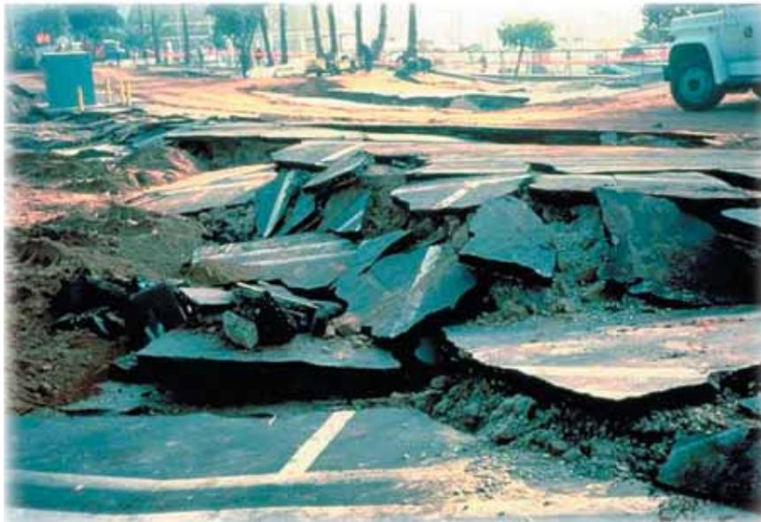
**Figure 3. This road was destroyed by liquefaction, when soil turned to liquid during the shaking of the ground. Many soils in the Seattle area can liquefy, including those in the Kent and Duwamish Valleys.**
