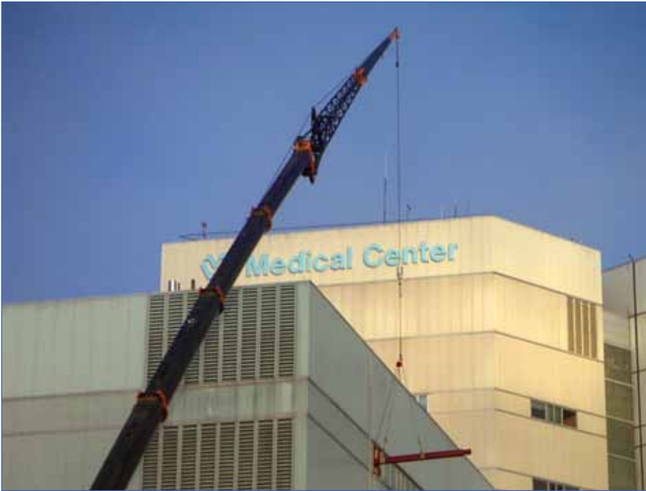
The Department of Veterans Affairs Hospital in Seattle provides both in- and out-patient care for thousands of veterans around the Northwest. A seismic evaluation of the hospital identified weak connections in the seismic bracing. An earthquake could have fractured the connections and endangered patients and staff. Seismic strengthening work was completed while the hospital was occupied and will allow the building to remain operational after an earthquake on the Seattle fault. Photo: Degenkolb Engineers
