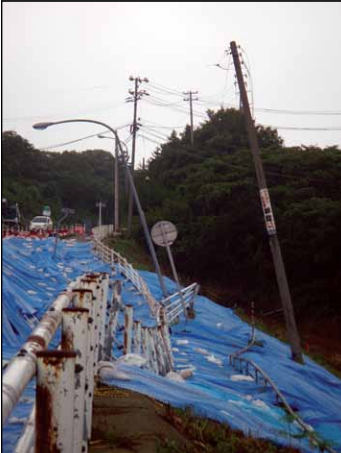
Landslides can be triggered by earthquakes that shake areas with water-saturated soils, a common occurrence in the rainy parts of Cascadia. They can block roads, but they can also disrupt utility lines, which may be more detrimental to the recovery of an area. The street light and utility pole in the picture above have both obviously been affected by this earthquake. Underground pipelines are not as easily seen but can also be affected. A buried water main and buried fiber optic main were both ruptured. Co-located lifelines can be interdependent and affect each other. Photo: Yumei Wang, DOGAMI
