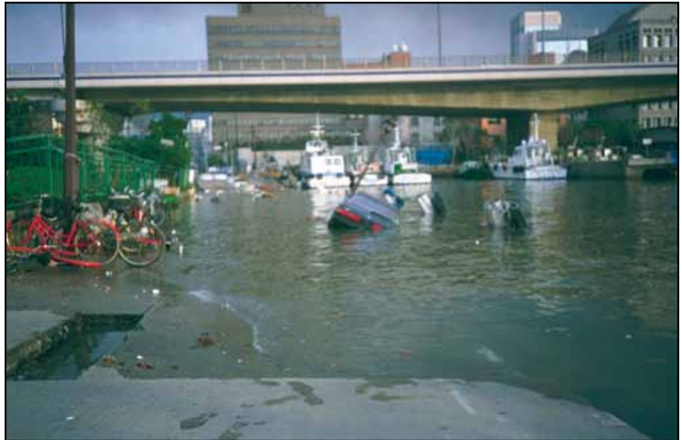
On January 17, 1995 a M6.9 earthquake occurred near Kobe, Japan. Cars, bikes, and buildings fell into the bay. Liquefaction and flooding were common near the waterfront. Areas like this can be designated parks, open spaces, or require special design and engineering. Photo credit: Dr. Roger Hutchison. Image provided by the National Geophysical Data Center
