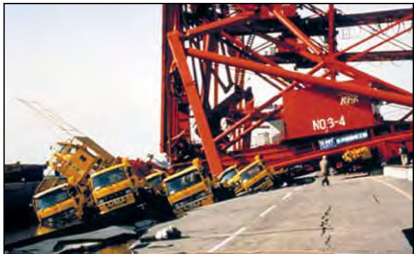
This crane, road to the port facilities, and numerous trucks were damaged by the M6.9 Kobe earthquake. Similar types of damage might be seen in Cascadia ports. Photo: EERI
