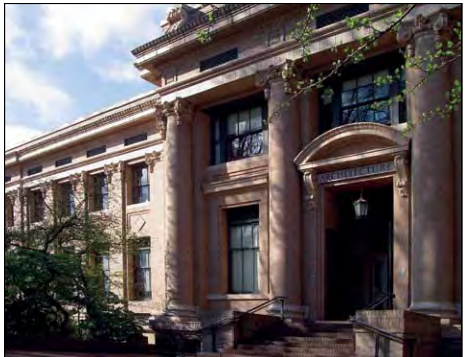
The University of Washington's Architecture Hall is one of the few remaining buildings from the Alaska-Yukon Pacific Exposition of 1908. As part of their Restore the Core program, UW is improving the seismic safety of their Seattle campus through systematic rehabilitation of older buildings. Strengthening work was performed from within the building to preserve its historic appearance. Photo: THA Architecture
