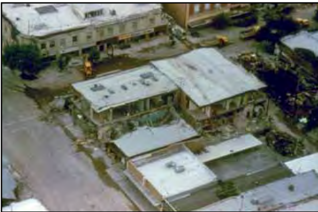
Some structures in Coalinga totally failed, while nearby buildings had only limited damage. In the upper right corner is a building destroyed by fire. Open fronts at street level a few blocks away had only glass breakage. Photo credit: Earthquake Engineering Research Institute (EERI)
