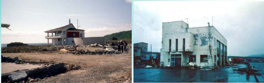
Figure 2-13 Examples of reinforced concrete structures that survived the 1993 Okushiri Tsunami: vista house at Cape Inaho (left); and fish market in Aonae (right).
